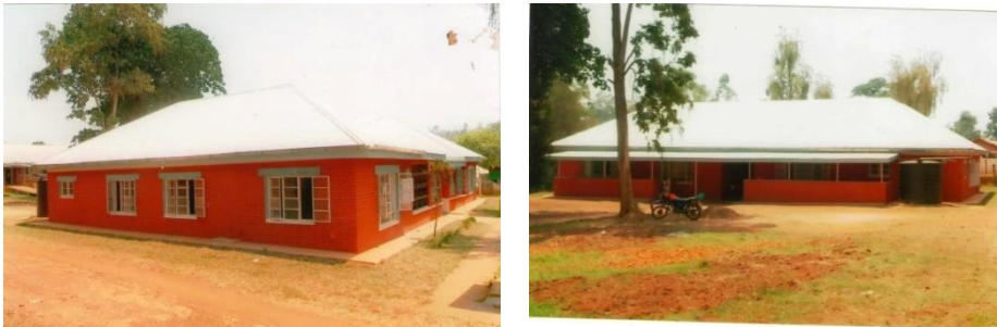
Plate 4: Two buildings completely renovated and equipped. Photo taken in December 2012.
