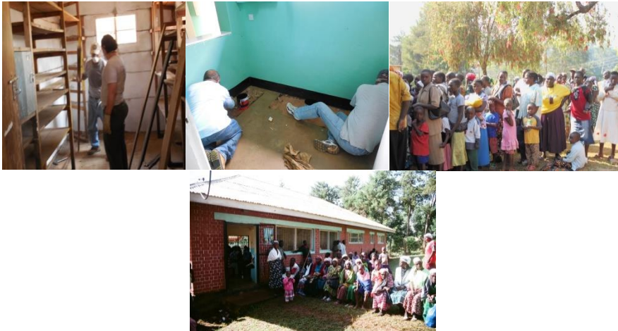
Plate 3: Renovation of Buildings and Medical Camps. Photos taken in August 2012
